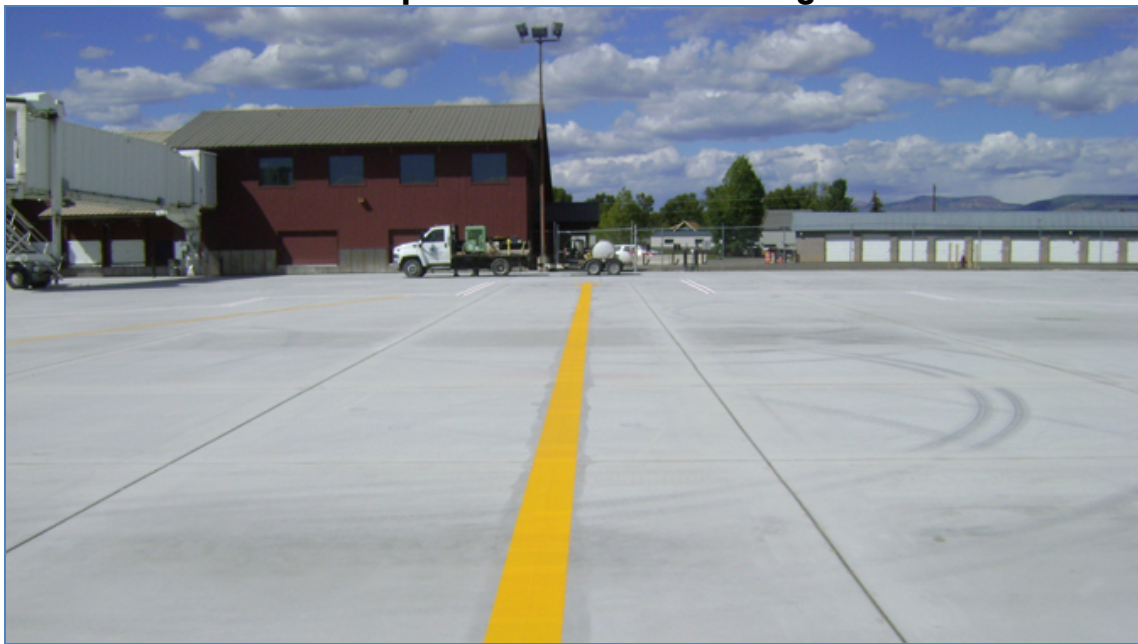
Ramp Side of Terminal Building
