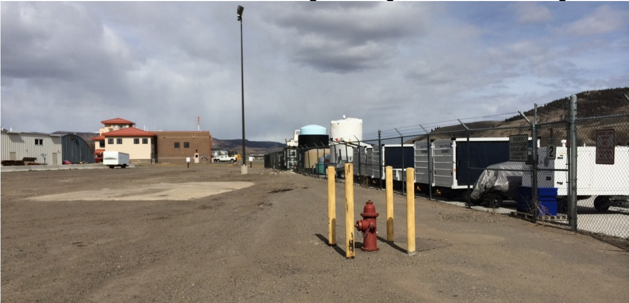
North from the Terminal Building - Looking Towards SRE Building
