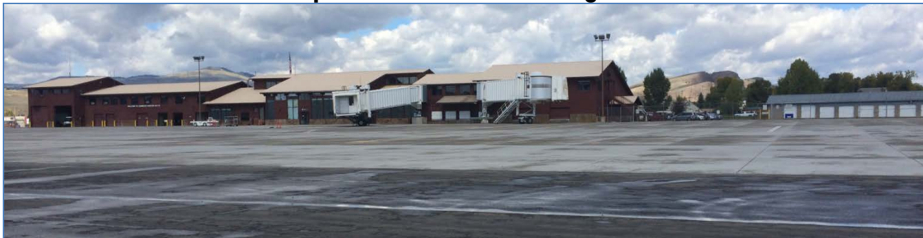
Ramp Side of Terminal Building
