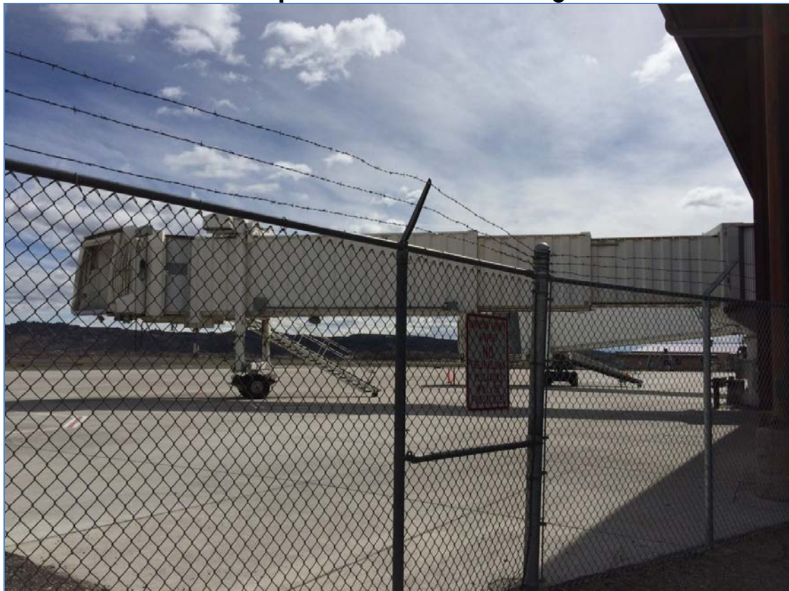
Passenger Loading Bridges Ramp Side of Terminal Building
