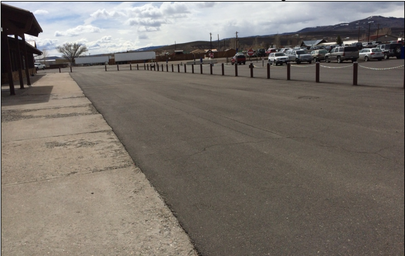
Terminal Curb Front and Vehicle Parking Lot
